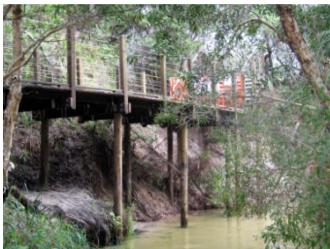
Other deteriorating Infrastructure
